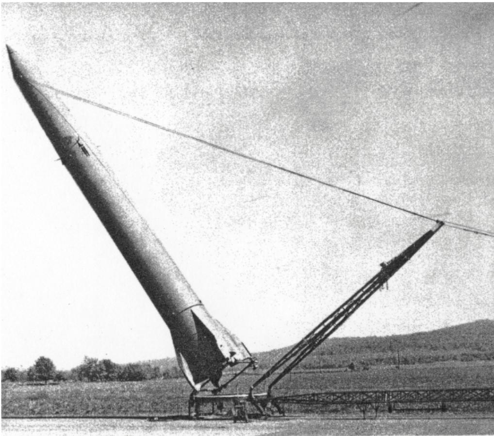
Figure 30. The missile is raised to the vertical position by the erector-servicer. The base of the missile is hinged to the launcher and the nose is raised to the vertical position by steel cables which are attached to the "A" frame.
